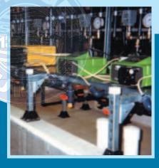
Ms. Joyce Kippen, Superintendent of the Ipswich, MA WTP has used Watson-Marlow Bredel tubing pumps for almost ten years in all of their chemical feed applications including sodium hypochlorite, alum and fluoride. "We have replaced all of our diaphragm pumps with tubing pumps as they offer SUPERIOR Reliability, accuracy and performance and do not vapor lock due to the off gassing of our hypo. Replacing the tubing takes only seconds and our maintenance costs have dropped to virtually zero."
